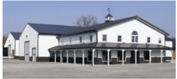
Ramco Supply Facility
